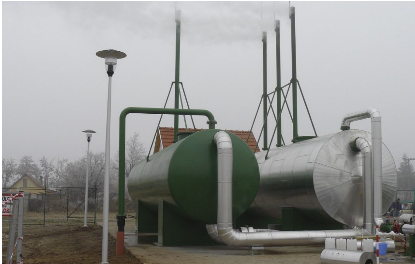
Production well and degassing buffer tank at the Makó cascaded system, Hungary
