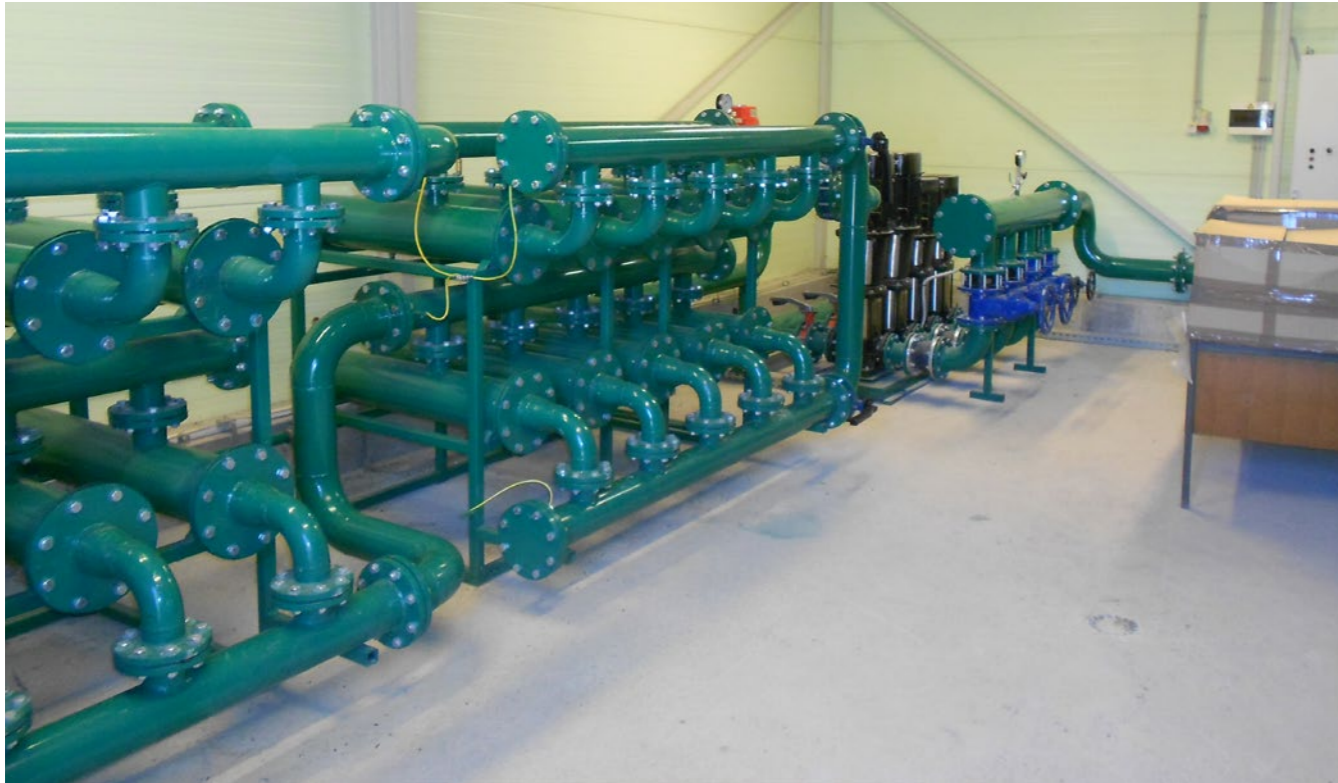
Filtering system prior to reinjection, Lendava, Slovenia
